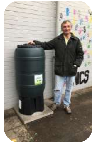
David connecting a water butt
